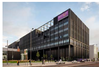
Manchester Engineering Campus Development, UK
